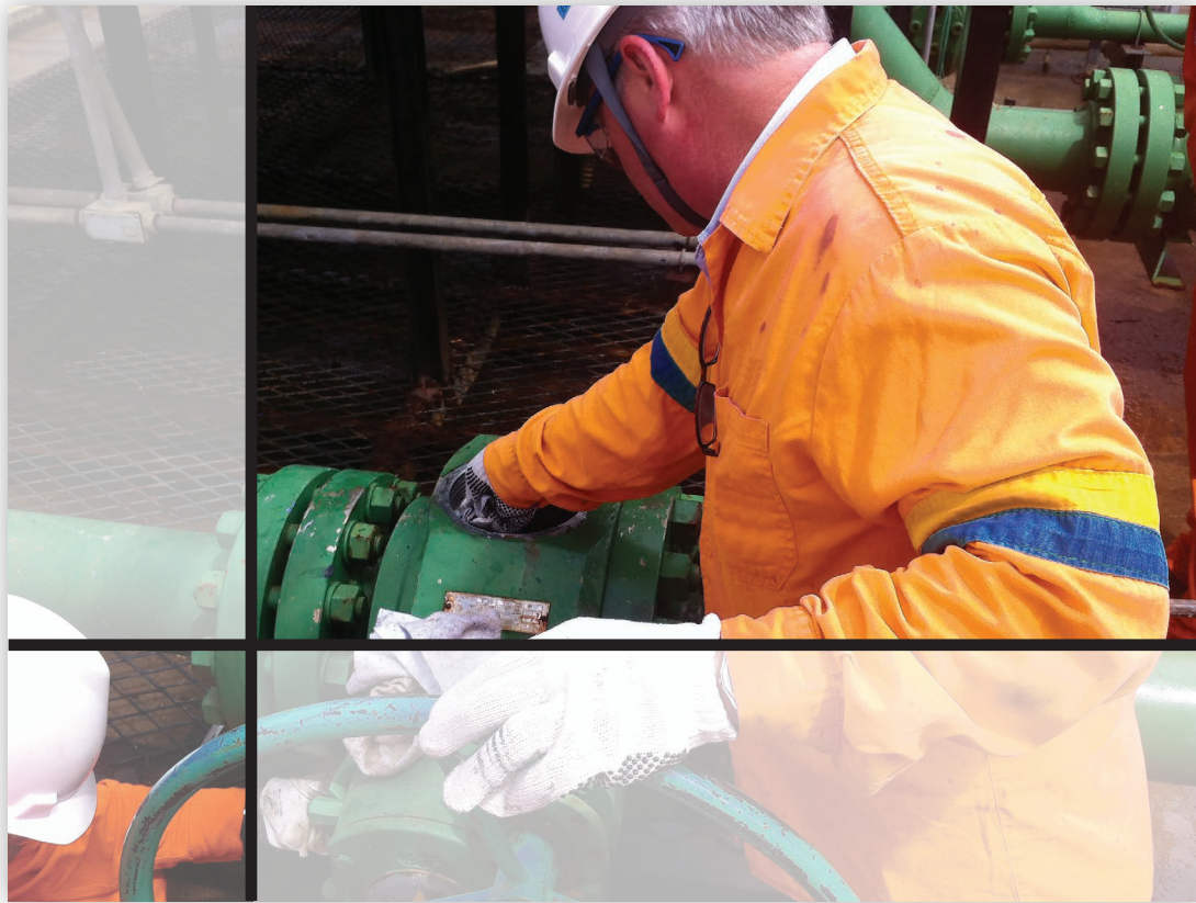
Training on site and Field Commissioning
